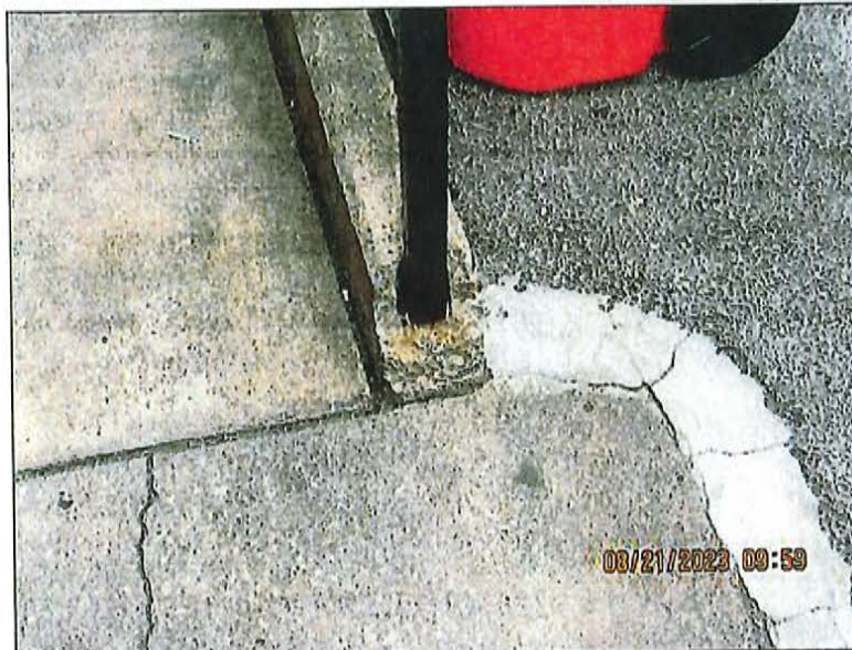
1.12 Item 5(Picture) Rear of building
