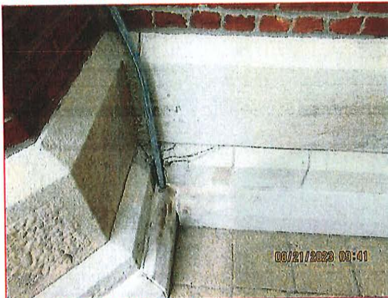
1.0 Item 5(Picture) Building Front
