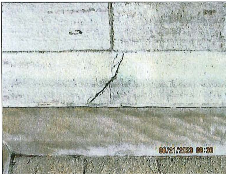
1.0 Item 3(Picture) Building Front
