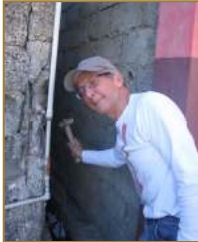
Jack Lydon inserting grounding rod
